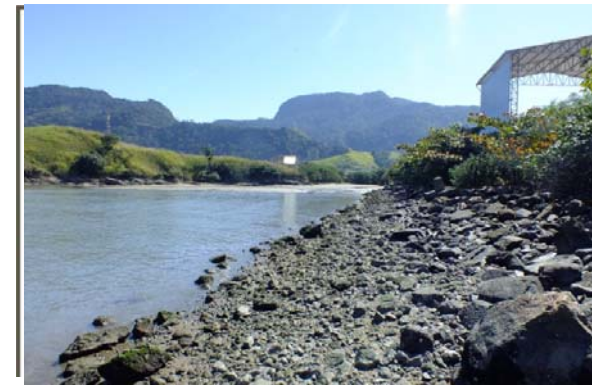
Rip rap view 2015
